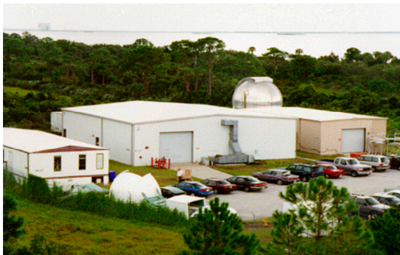
Fig. 2: A bird’s eye-view of the ISTEF, showing the laser laboratory and the dome containing the transmitter and receiver.
